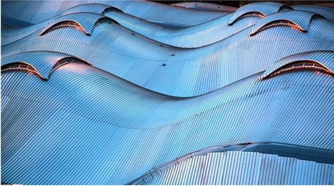
**Fig. 2** The Southern Cross Station in Melbourne, Australia covered with straight metal strips (from flickr.com).
